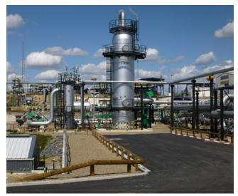
The project took nine months to complete, from award to commissioning, and involved upgrading the units of gas treatment by adding a column of dehydration and its separator downstream to increase the site's processing capacity.
