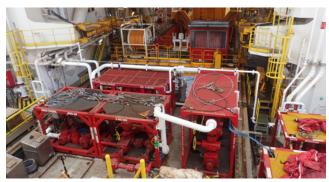
Additional fully pre-fabricated structures for the umbilical reels on the Xmas tree trolley, along with detailed engineering and positioning of equipment on the deck, allowed a minimal impact on the structural modifications during the installation.
