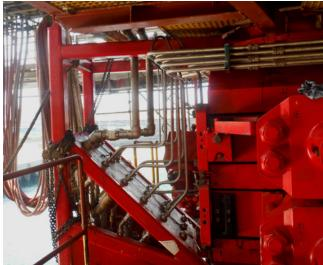
The UMW Naga 8 is a jack-up rig drilling in the northeast of Malaysia. The rig and operators requested a few upgrades to adapt it for the high-pressure and high temperature (HPHT). This involved the addition of a new kill-and-choke line inlet and outlet on the blowout preventer (BOP). This resulted in the requirement to install additional Koomey lines to operate the new valves as well as re-routing of the BOP tubing to make space for the new valves assembly.
