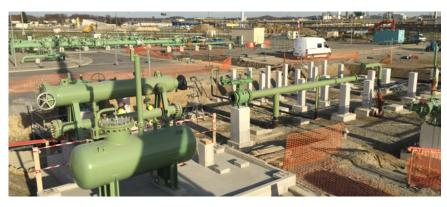
This difficult multi-discipline project is a new challenge for 3C Metal and its partners. The RZL project will divert the main gas interconnections, operated by TIGF, from the former Total gas factory in the area. This 18 month project includes the construction of six main pipelines, four horizontal drilling operations of 40m long, two horizontal directional drilling
