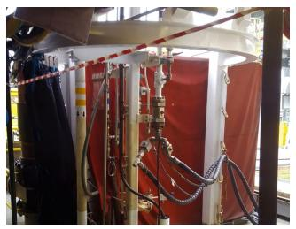
Ensco requested further preventive measures for semisubmersible ENSCO 8504 by having blast curtains installed by 3C Metal. The blast curtains are designed to stop any projectiles caused by the unlikely event of a high pressure failure in the area of the drill floor. 3C Metal selected a suitable curtain designed to absorb the energy from a high pressure failure. 3C Metal was responsible for the design, fabrication
