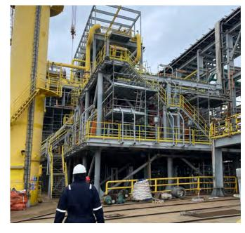
3C Metal conducted a comprehensive site survey to identify the missing lifting points on the process modules. Based on the findings, a detailed execution plan was developed for the removal of existing insert portions and their replacement with prefabricated lifting padeyes — a strategy specifically designed to minimize onboard fabrication activities.
